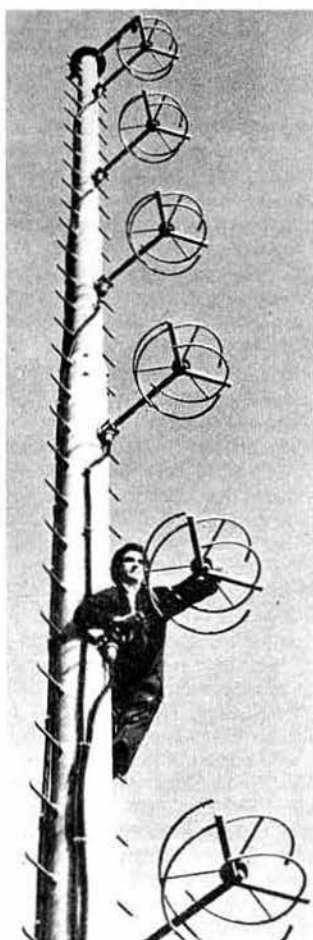
Stack of six circularly-polarized Band 2 elements forming the broadcasting antenna used by the IBA at Croydon for Capital Radio and LBC
